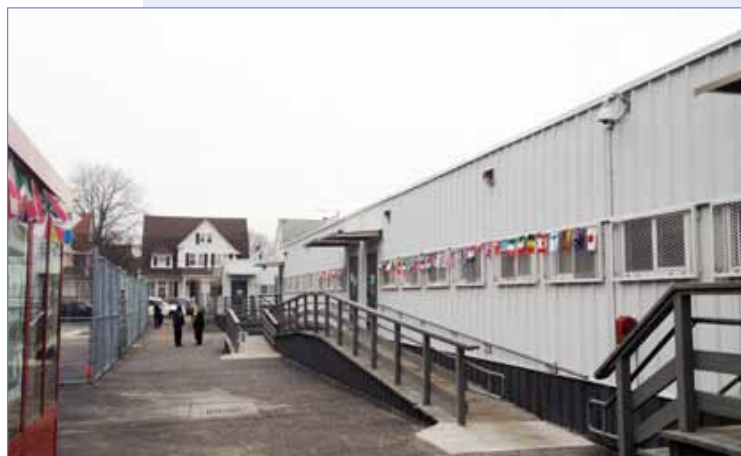
Temporary Classroom Units at Richmond Hill High School
